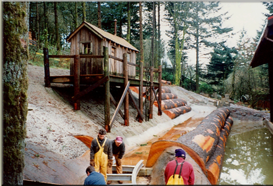
Construction Big Timber Log Ride
