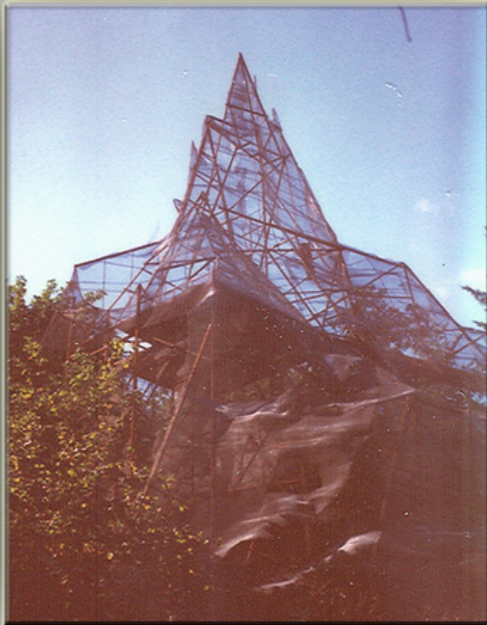
Construction Ice Mountain
